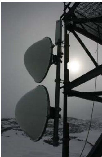
3 ft. antenna deployed along an oil pipeline in the Middle East
